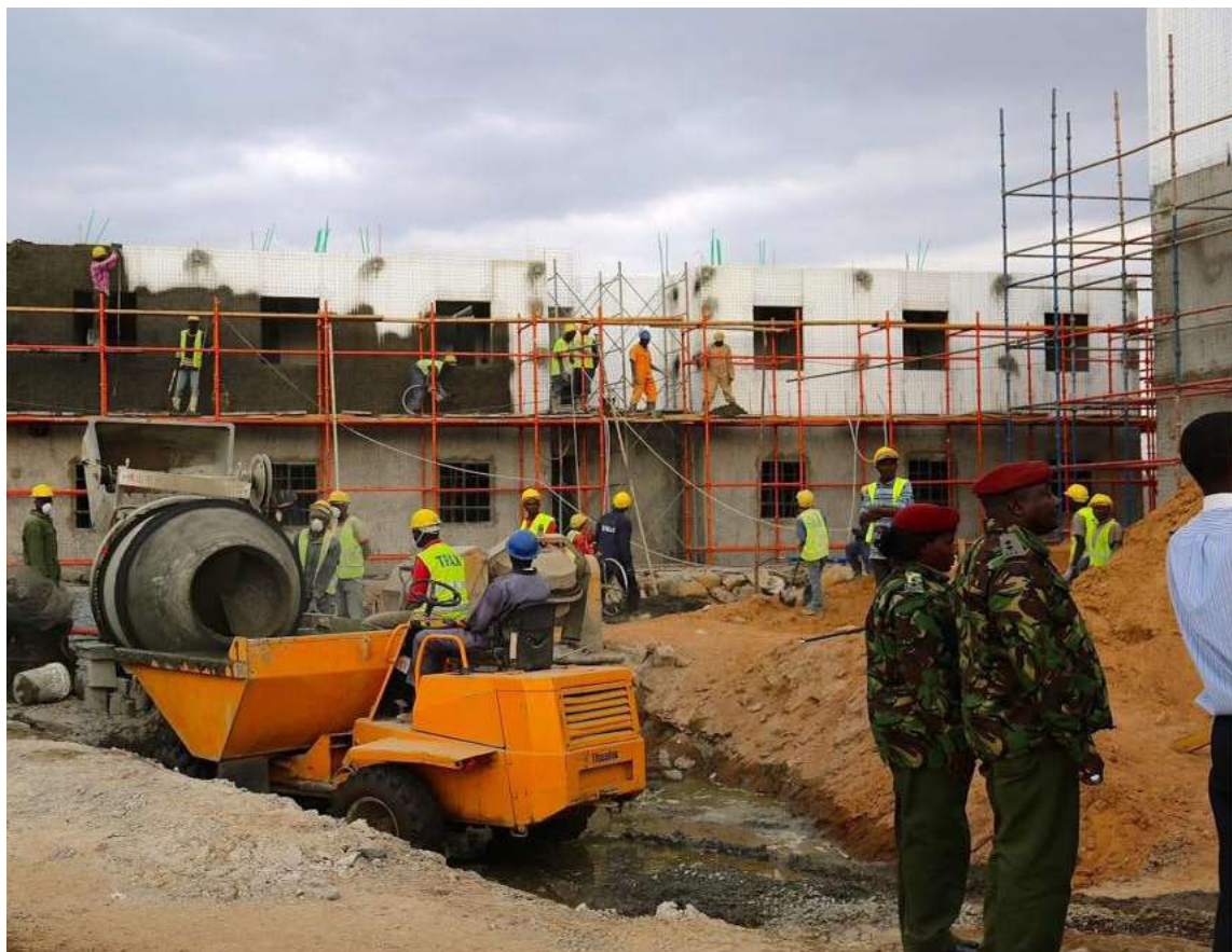
Construction of Police housing units in Ruiru, Kiambu County
