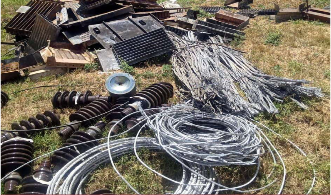
Vandalized Kenya Power transformers, rolls of aluminum and conductors recovered in Juja Area, Kiambu County
