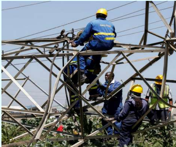
Kenya Power and Lighting Company officers repairing a vandalized pylon.
