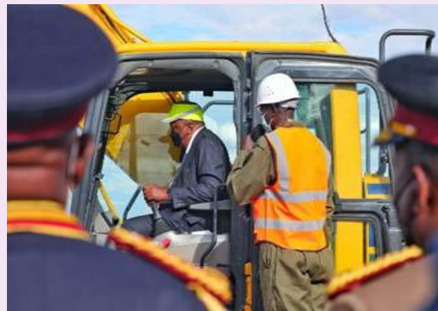
H.E The President during the ground breaking of NPS Referral Hospital at Mbagathi, Nairobi
